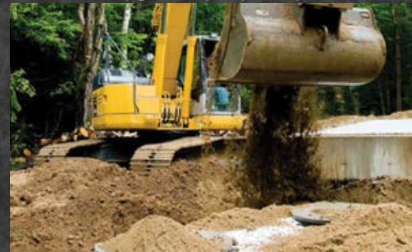
septic system installation backfill | grading
